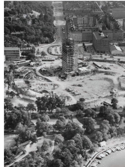
Figure 1. Construction of Wenner-Gren Center. Source: Oscar Bladh and Stadsmuseet
