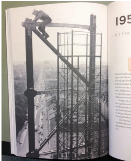
Figure 2. Scaffolding. Source: Harry Dittmer and Nordic Photos
