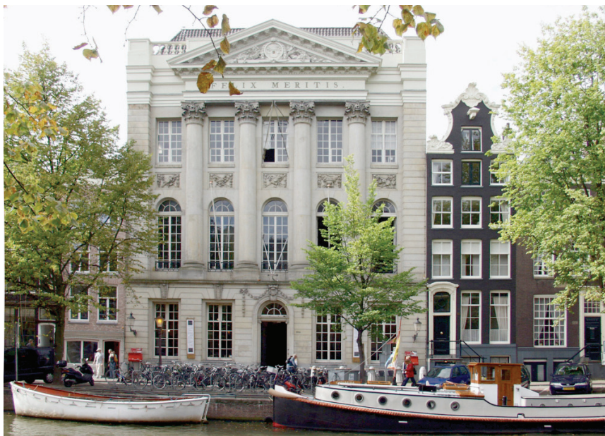
Figure 1. Facade of Felix Meritis, Keizersgracht 324, Amsterdam. Source: Author's photograph.
