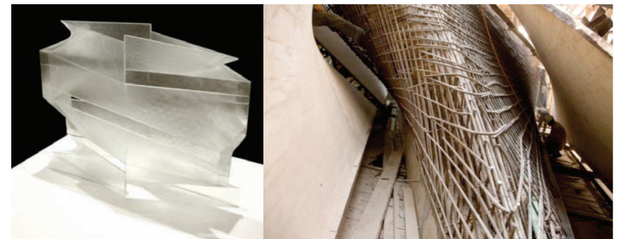
Figure 1. The lightfall: Conceptual model, right. Preparation of wooden formwork and steel reinforcement bars, left. Source: The Tel Aviv Museum of Art.
