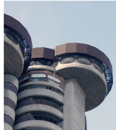
Figure 2: Detail of the visual transition element between the outer vertical slabs and the discs of the social core. Source: Photograph by the author, 2011
