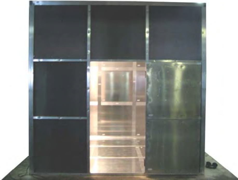
Figure 119 Shielding on all the sides of the substation (Conf. 4)
