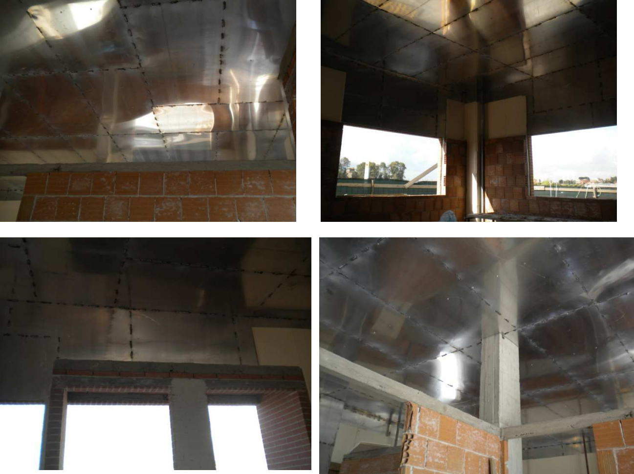
Figure 143 – Pictures of the conductive shield during the realization of the system
