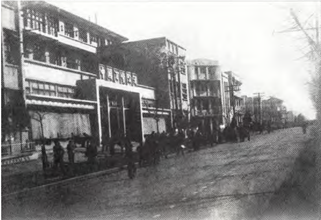
Figure 25 Wuyi Avenue West Constructed in 1952
