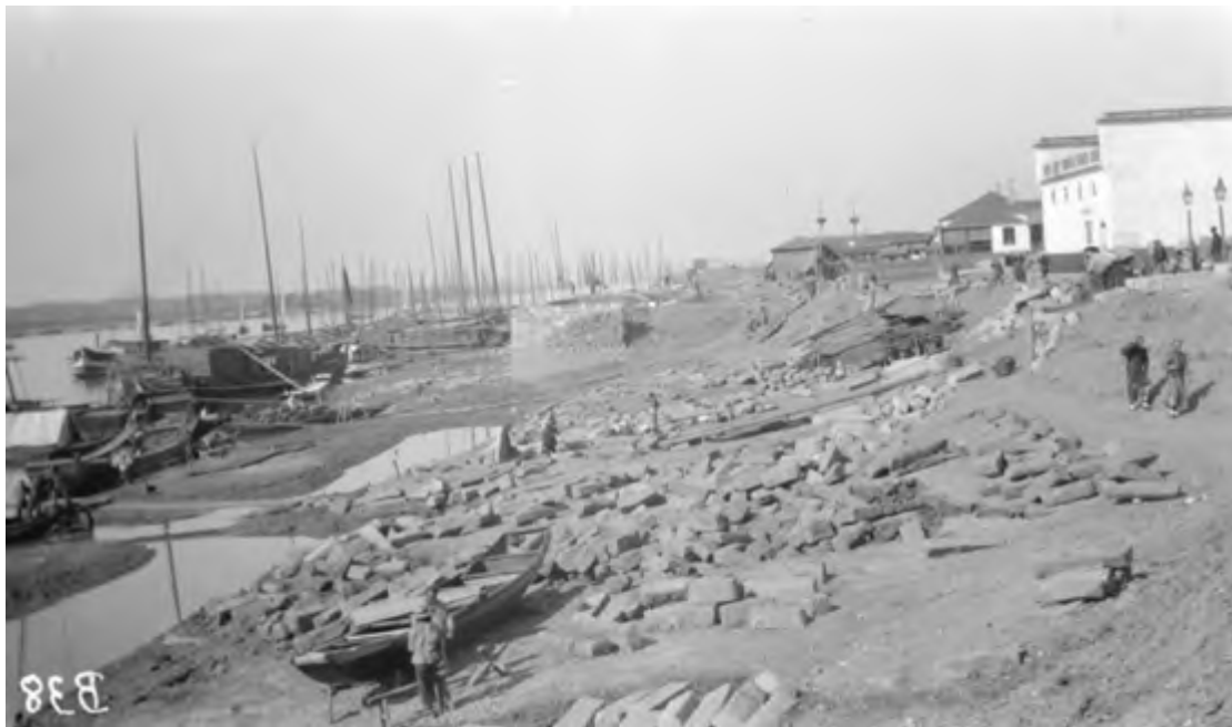
Figure 16 Bund Construction in Changsha 1906-1907
