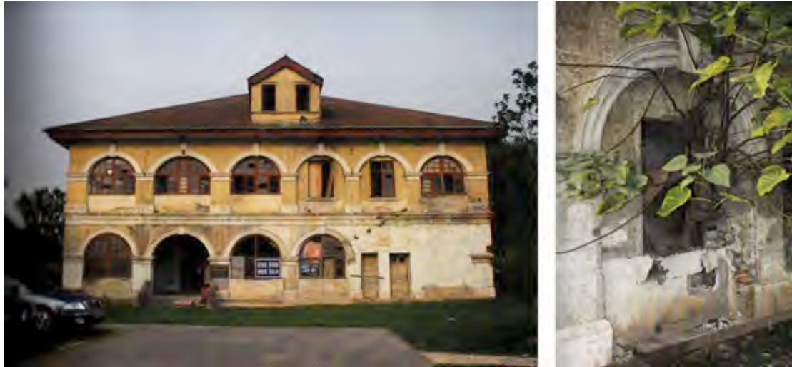
Figure 91 Former Site of Changsha Customs Office in Need of Restoration
