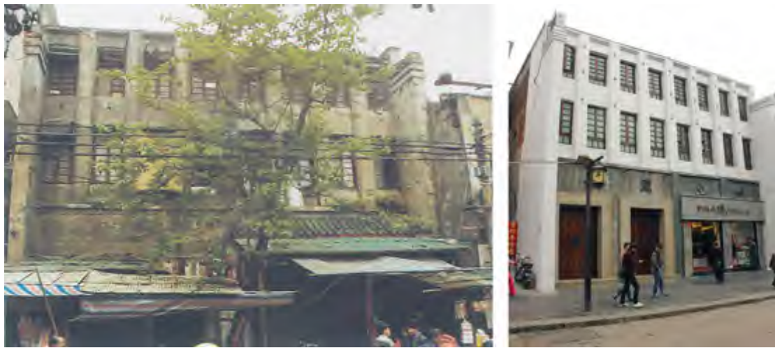
Figure 48 Lisheng Store (利生盐号) in Taiping Street in 1990s and 2013
