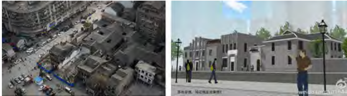
Figure 112 Suzhou Hall and Hong Financial House before Dismantlement and Rendering for Relocation Project
