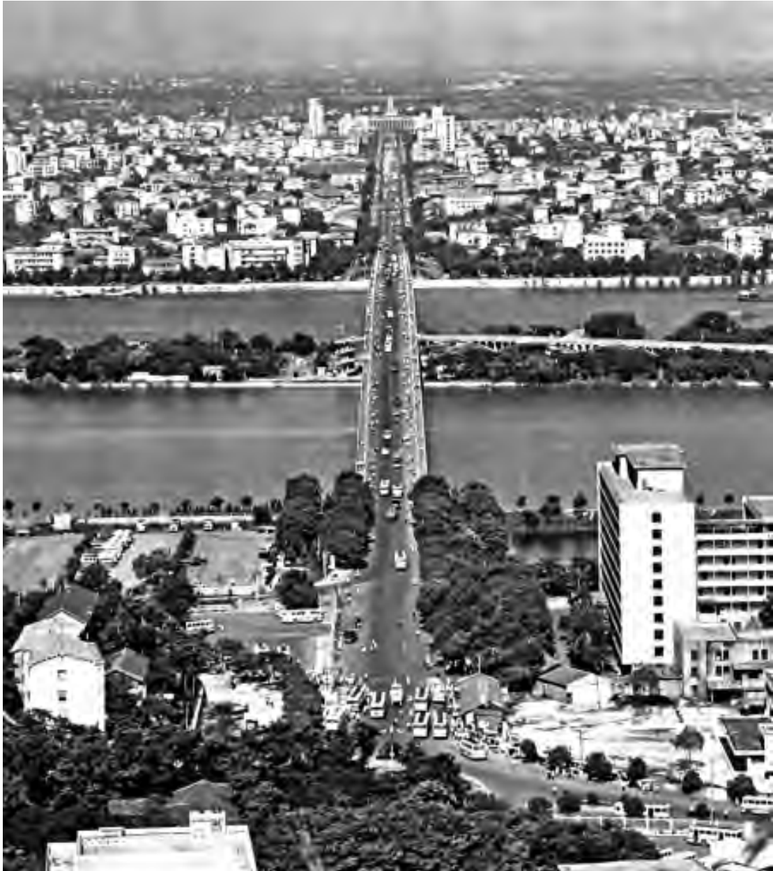
Figure 29 Axis of Relocated Changsha Train Station, Wuyi Avenue and Xiangjiang Bridge (Juzizhou Bridge) in 1983
