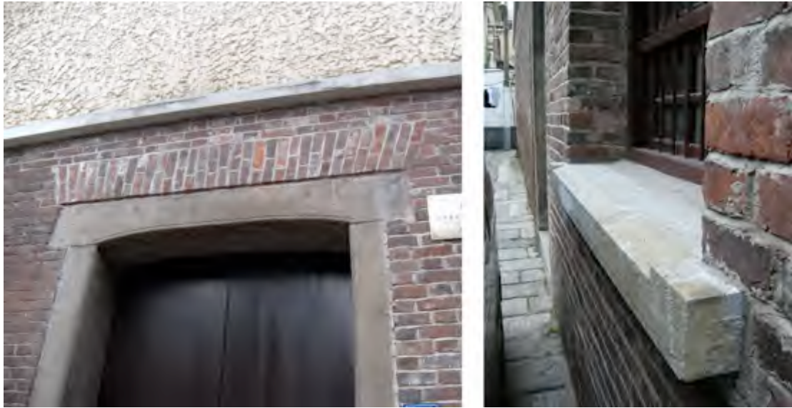
Figure 89 Beam on Entrance and Windowsill After Restoration
