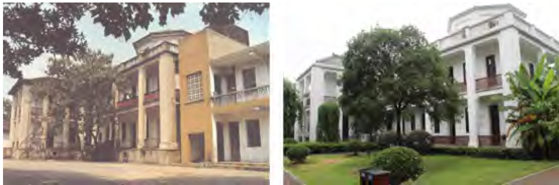
Figure 109 Former Residence of Tang Shengzhi on Juzhou Island Before and After Restoration in 2009
