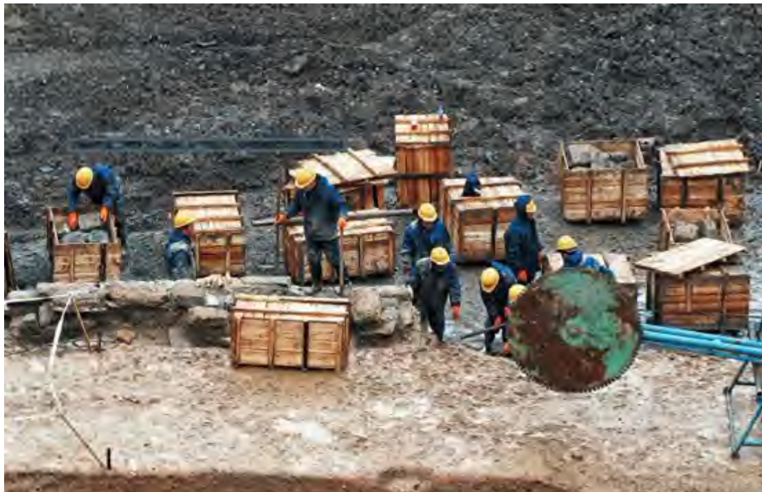
Figure 101 Dismantling the Piece of City Wall
