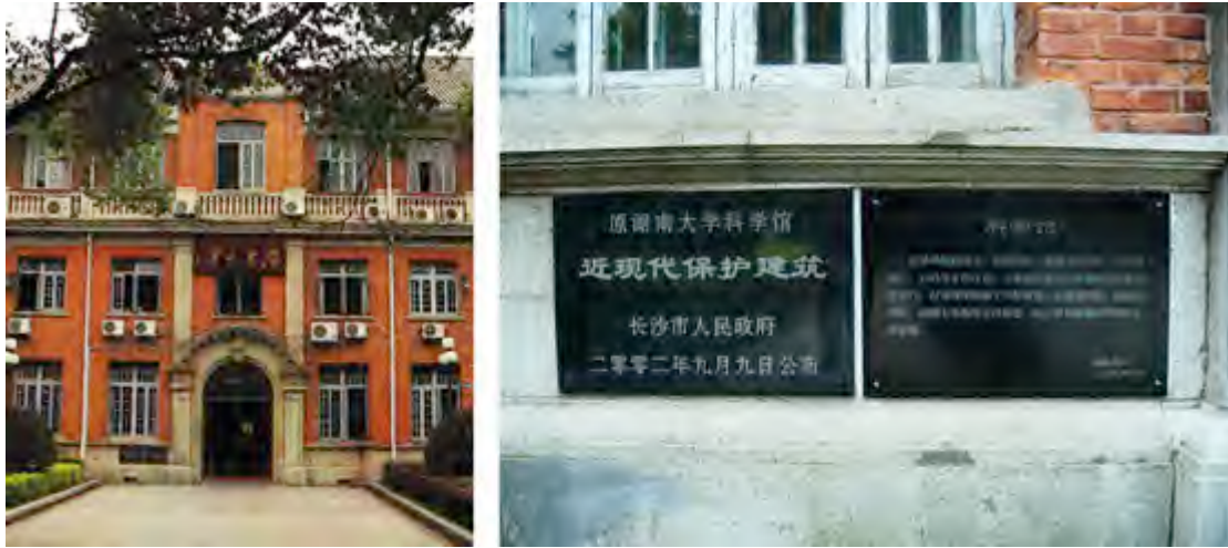
Figure 42 Declaring and Illustrative Plaques on Facade of 4-18 Kexue Building in Hunan University
