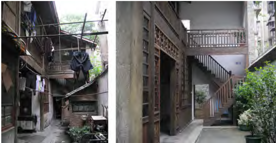
Figure 110 Former Shelter of Jin Jiu before and after Restoration in 2009
