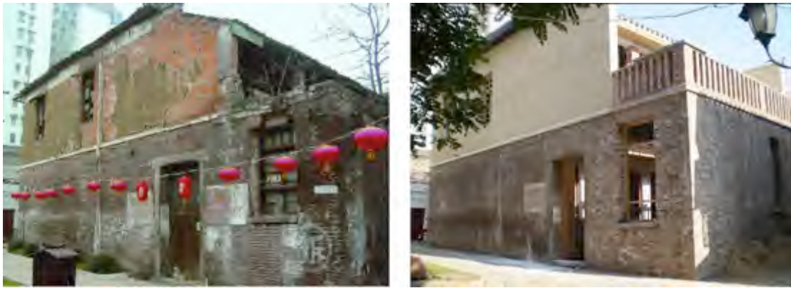
Figure 88 Former Residence of Cheng Qian Before and After Restoration in 2011
