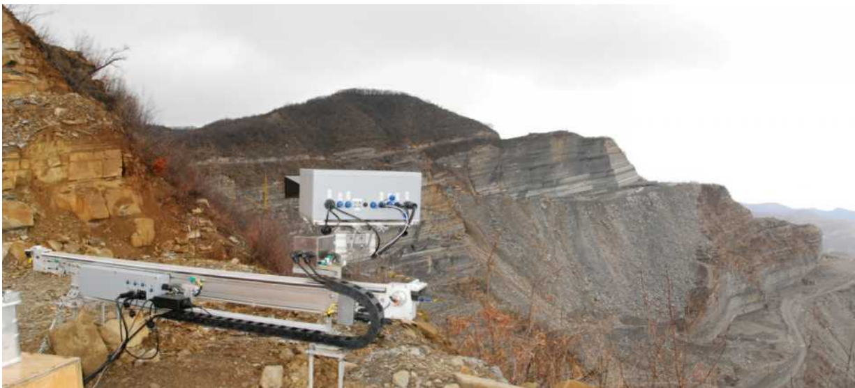
Figure 6. GBInSAR installation at the sandstone ('pietra serena') quarry in Firenzuola (Firenze - Italy)
