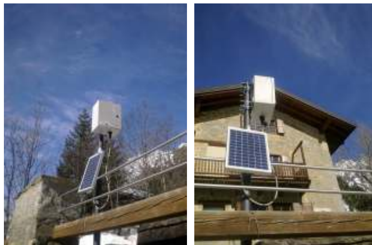
Figure 6.14. Experimental installation of the first GPS network node GP01.
