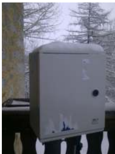
Figure 6.15. Experimental installation of the first GPS network node GP02.
