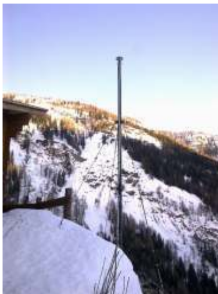
Figure 6.13. Antenna of the permanent station FOND (the receiver is inside the building of Fondazione Montagna Sicura).
