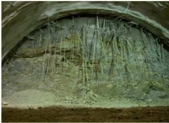
Fig. 2. Tunnel face (intensively weathered mica schists)
