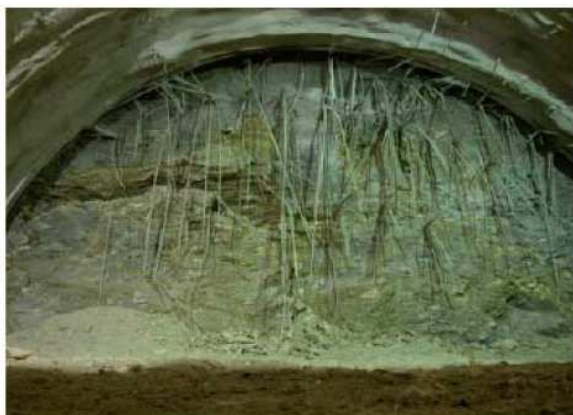
Fig. 2. Tunnel face (intensively weathered mica schists)
