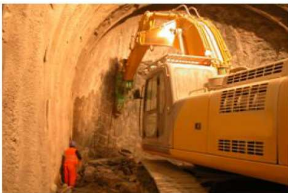
Fig. 4. High Hydraulic Energy Hammer at work while a second worker provides the machine operator with visual help and “tries” to reduce the airborne dust pollution by spraying water onto the face
