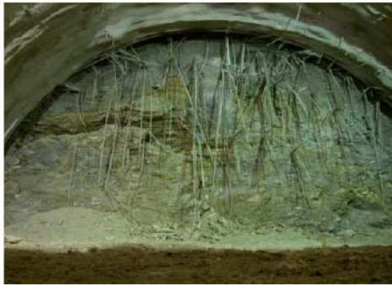
Fig. 2. Tunnel face (intensively weathered mica schists)
