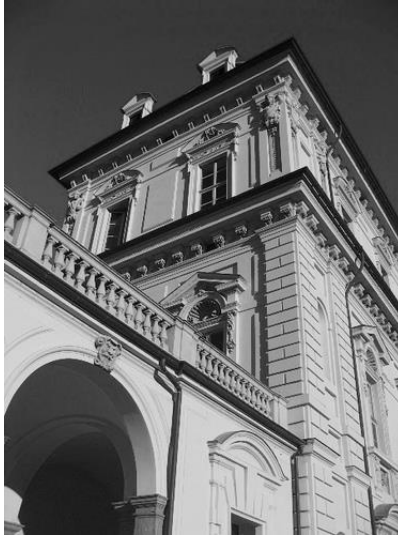
Figure 9-3: Uniform look after the restoration
