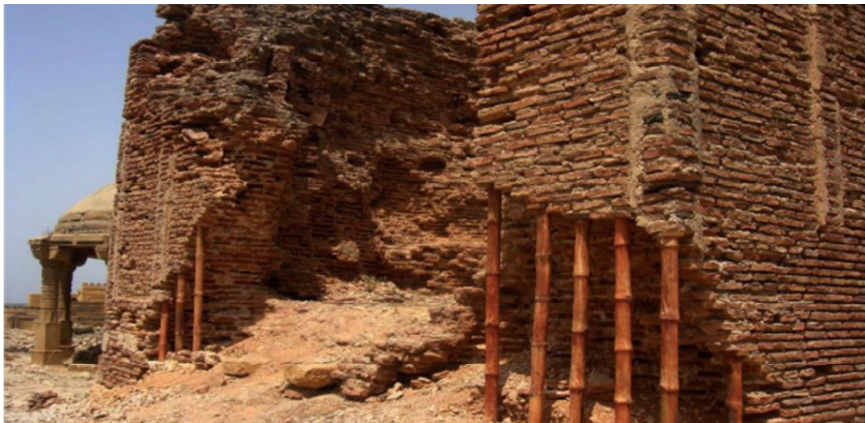
Figure 9-11: The underpinning activity executed on site
