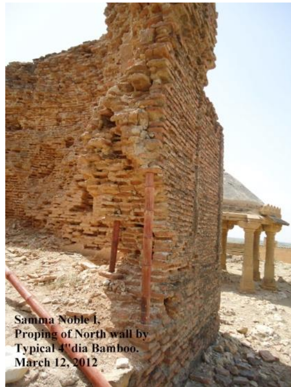
Figure 9-12: The side views of underpinning activity
