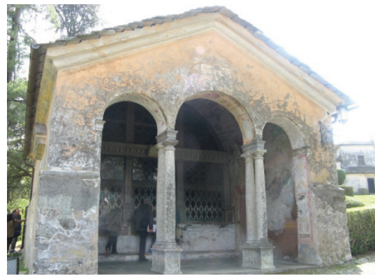
Fig. 4 Decay of historical plasters because of the rain infiltrations (Chapel n. 13—The Temptations).
