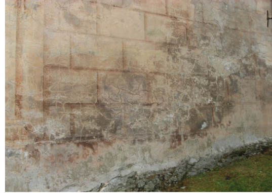
Fig. 3 Delamination and detachment of artistic plasters because of the rising damp effects due to capillary action or rain infiltration (Chapel n. 23—Jesus is taken).
