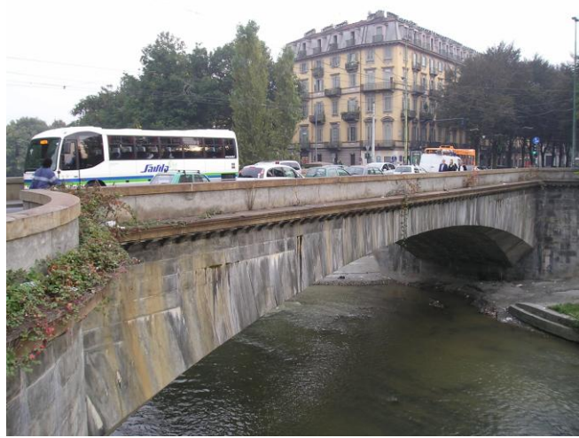
Figure 11. Mosca Bridge under Service Loads.
