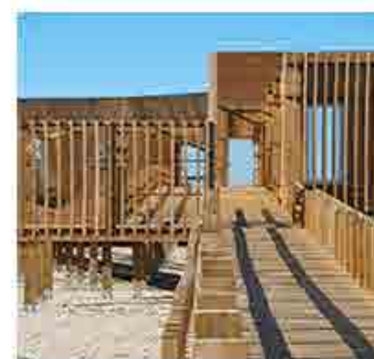
EVOA - Environmental Interpretation Center, Mair Arquitectos (Portugal)
