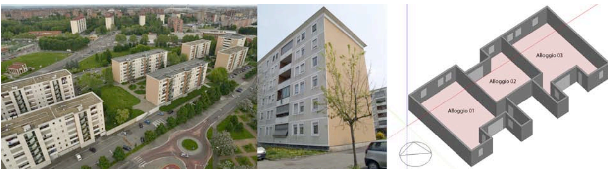
Fig 1: 4 Naturwall Case study model. Located in via Pietro Cossa in Turin. On the right the plan of the main floor.
