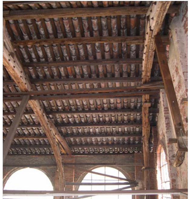
Figure 6 – The former Trombetta wool mill, Biella. Detail of the unstable arches. (photo Mattone).
