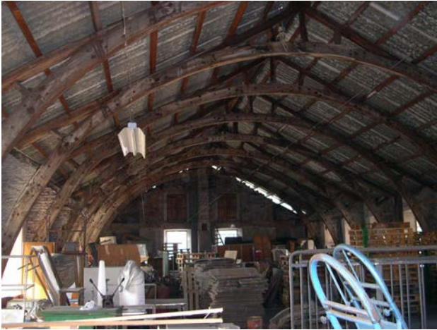
Figure 7 – The former Gallo wool mill, Sagliano Micca (Biella). The wooden arch structure. (photo Mattone).
