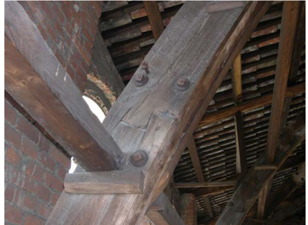
Figure 5 – The former Trombetta wool mill, Biella. Detail of the arches. (photo Mattone).
