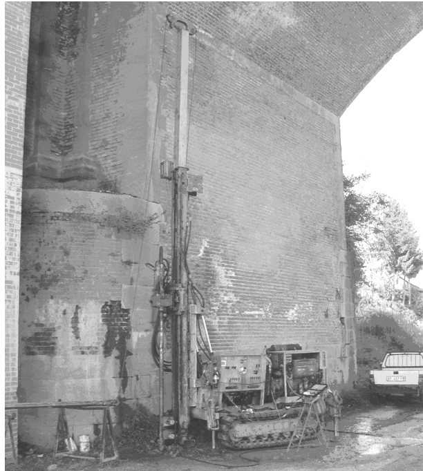
Fig. 3. Drilling equipment used for the core destruction monitoring drilling on the shoulder of the bridge over the Gesso Stream at Cuneo
