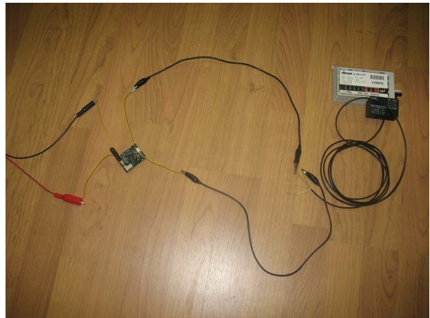
Figure 6. Smart grid node during the massive stress test connected to commercial pulse generator which will be connected to the gas meter in a real application.
