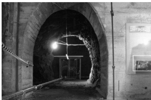
Figure 5. View of one of the vacuum pipes hosting the laser beam of a ring-laser in the Cashmere cavern near Christchurch, NZ.
