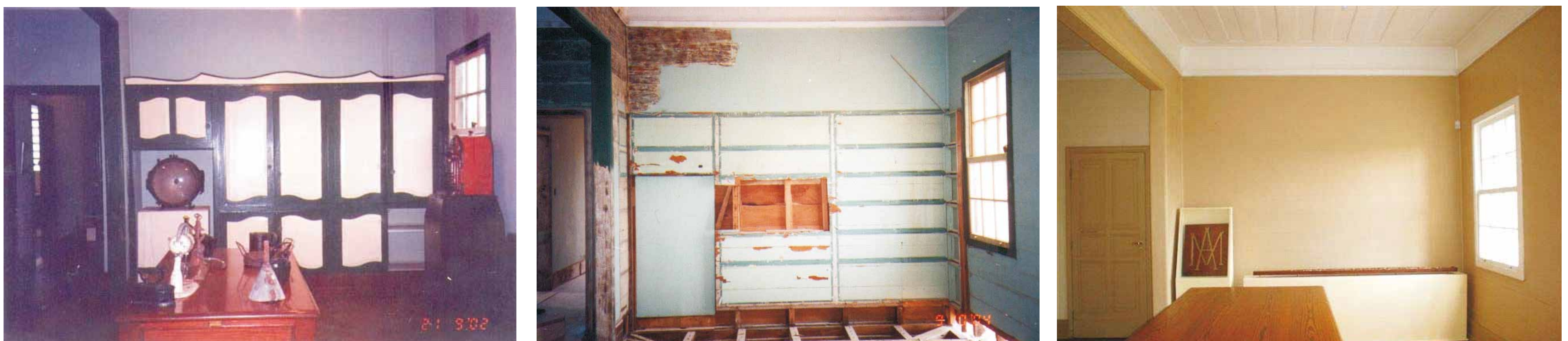
Ambient: pantry. Before, (2002). During, (2004) and after (2012)
