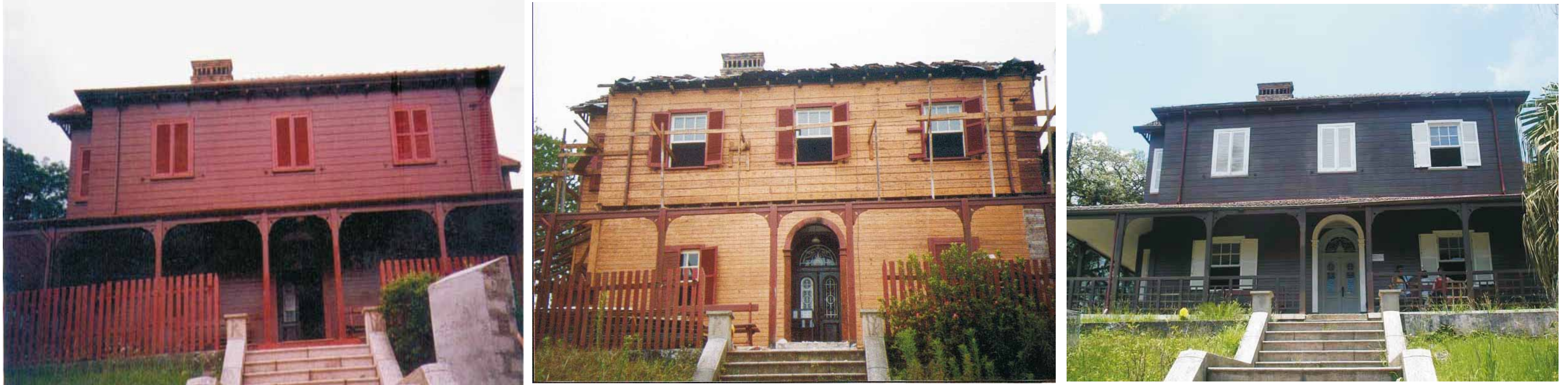
Main Facade. Before, (2002). During, (2004) and after (2012)
