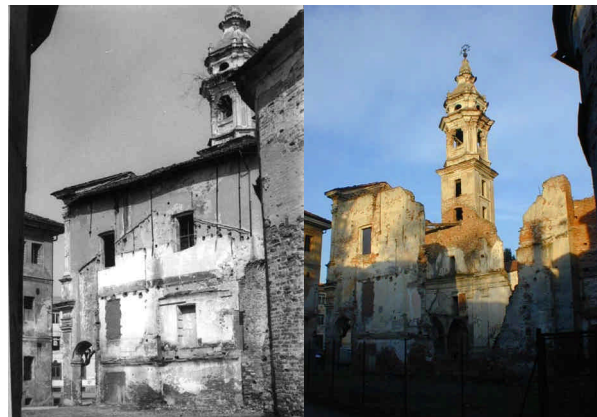
Figure 2. The church before and after the damage of 1984
