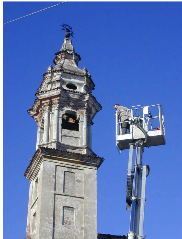
Figure 3. Photogrammetric taken of the bell tower
