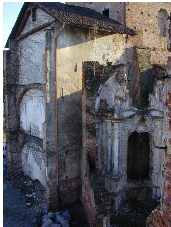
Figure 3. Rests of the vaults
