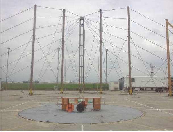
Figure 2. In the background, Alenia Aermacchi's inverted-V antenna and, in the foreground, the table supporting the cable harness (Copyright @Alenia Aermacchi)
