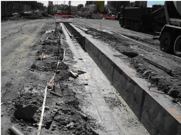
Figure 5. View of the short trench made initially to allow excavation of a panel in order to begin the construction of concrete diaphragm walls.
