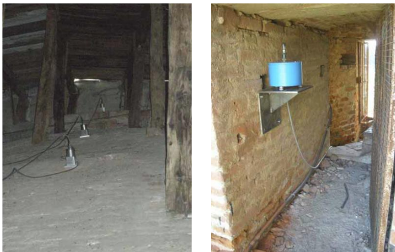
Figure 4.17 - Examples of accelerometers and geophones placement: (a) on the top of the dome and (b) on a column.
