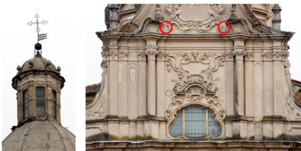
Figure 4.31 - (a) The lantern (b) The jut of the façade and the instrumented locations.
