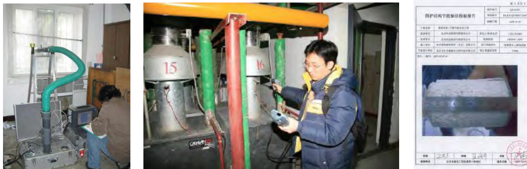
Fig. 6.48 Work photo and document of regular check
