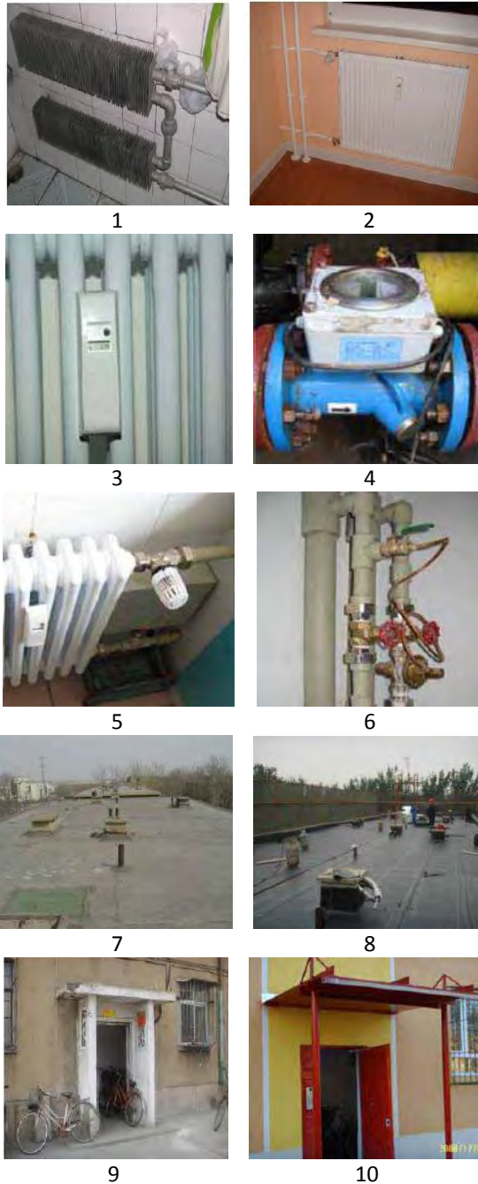
1. Heat radiator before refurbishment 2. Heat radiator after refurbishment 3. Electronic heat distribution meter 4. Ultrasonic heat meter 5. Binary thermal control valve 6. Self-operated differential pressure controlling valve 7. Roof before refurbishment without insulation 8. Roof after refurbishment added insulation layer (14cm PU or XPS ) 9. Building entrance before refurbishment 10. Building entrance after refurbishment
