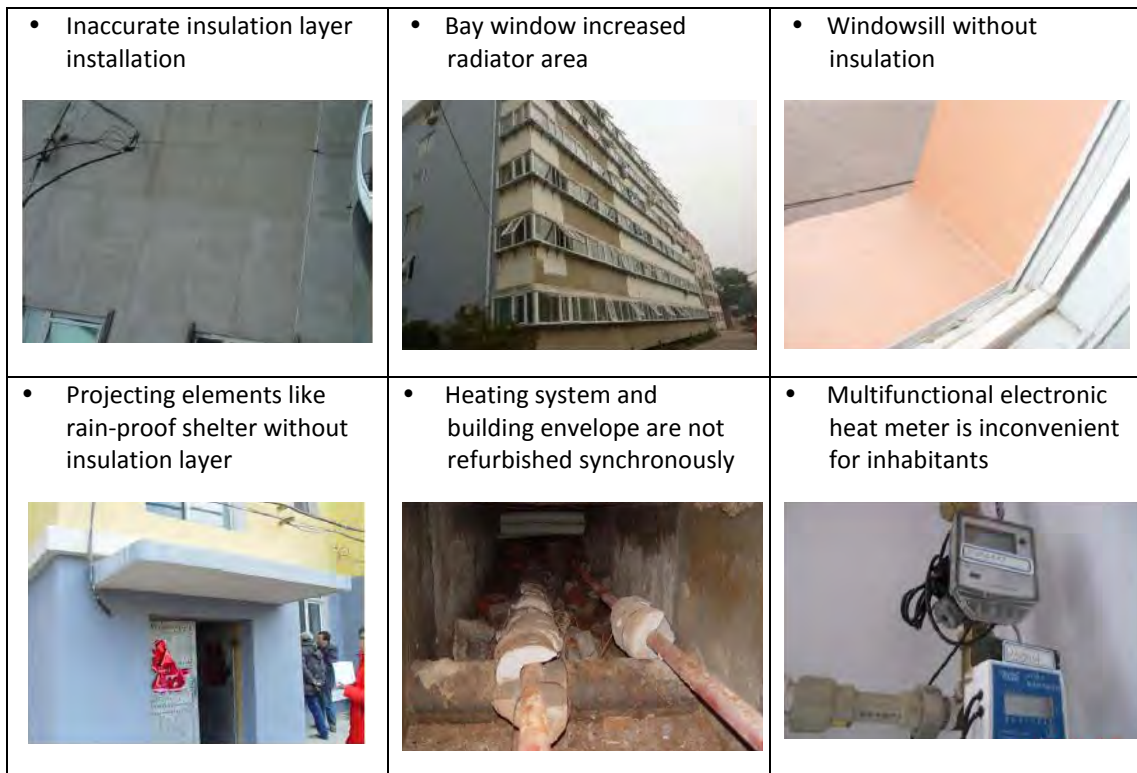
Fig. 6.7 Common design problems in residential building refurbishment project in China
