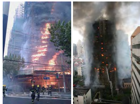
Fig. 6.5 Photos of Shanghai residential building accident 2010 Nov.15 th http://www.flickr.com/photos/cpj/5178106136/
