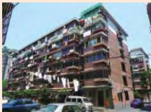
Fig. 6.21 Photo of case study 3 Top: Before refurbishment Bottom: After refurbishment
