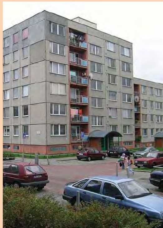
Fig. 3.12 Photo of Project in Haviřov before refurbishment
