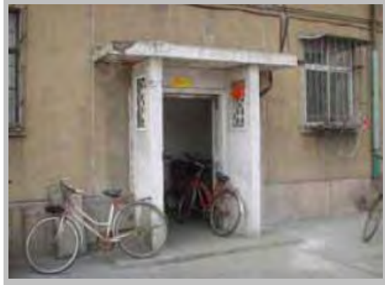
Fig. 6. 10 Photos of existing building before refurbishment
