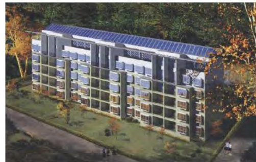
Fig. 4.9 A typical building integration photovoltaic system with shading materials.
