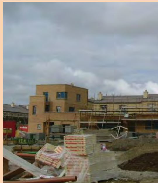
Fig 3.11 Photo of Project in Dublin before refurbishment
