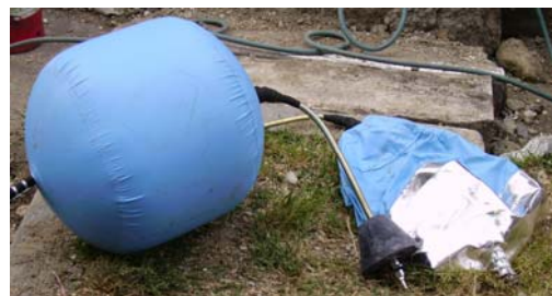
Fig. 2 Blocking balloons with frustum of cone plugs to stop the pipe holes; the deflated balloon is strengthened by an aluminium sheet which constitutes a protection against sparks originated by welding operations.
