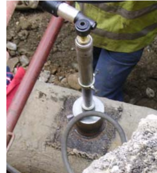
Fig. 1 of the pipe-boring machine and of the collar on a steel pipe
