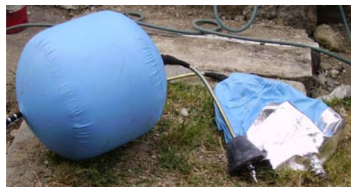
Fig. 2 Blocking balloons with frustum of cone plugs to stop the pipe holes; the deflated balloon is strengthened by an aluminium sheet which constitutes a protection against sparks originated by welding operations.
