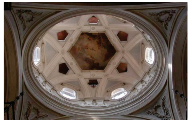
Fig. 3 - Removal of the various paint layers;
