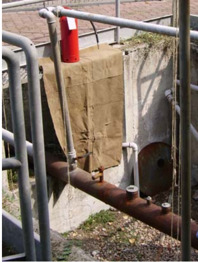
Fig. 4 Trench and pipe in test area.
