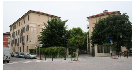
Fig. 1. Overview of Arquata Social Houses in Torino.
