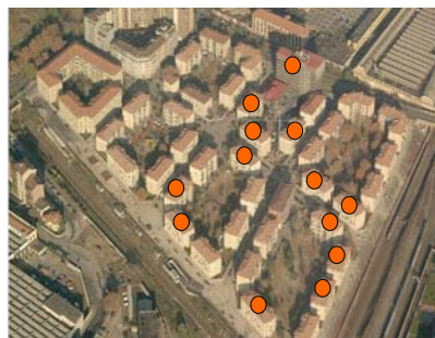
Fig. 3 Arquata district and ATC building PV panels.
