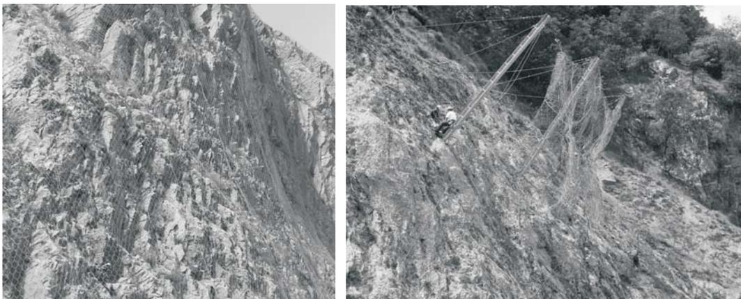
Fig. 6. Details of the drapery wire meshes and net fences installed on the rock slopes to protect the quarry yard
