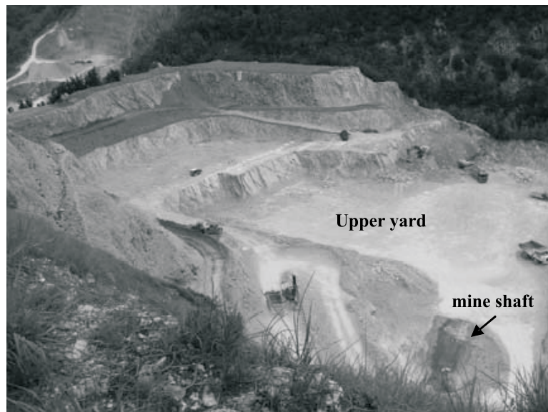
Fig. 5. Overall view of the limestone quarry
