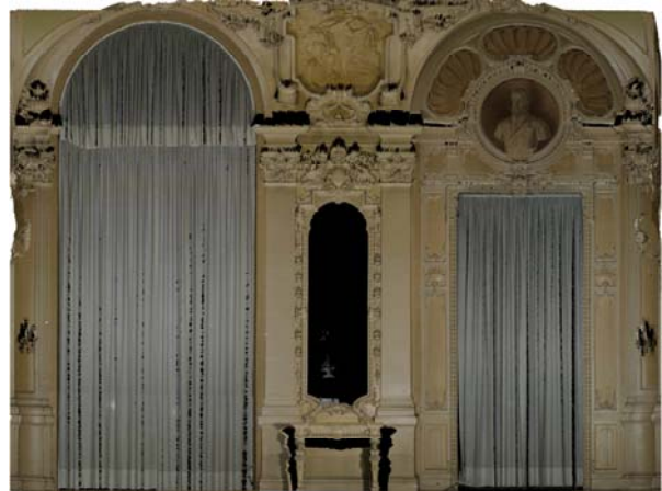
Fig. 9 – The true orthophoto of the western wall.
