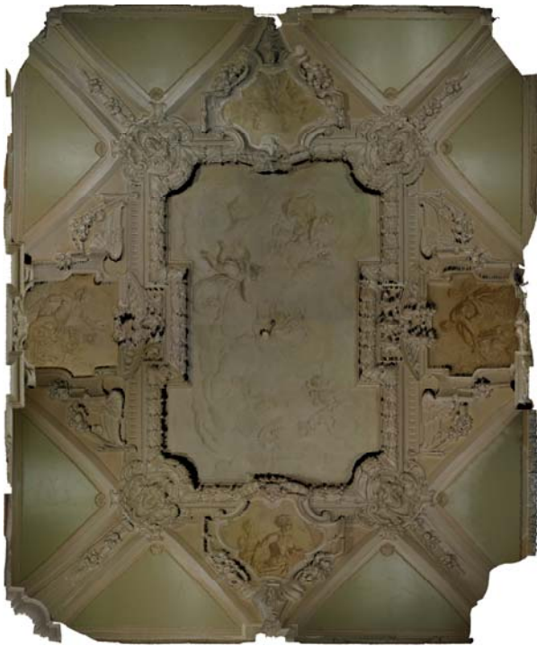
Fig. 11 – The true orthophoto of the ceiling.
