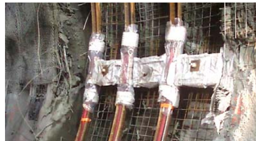
Figure 3. Highly Deformable Concrete (HiDCon) elements during installation between the TH steel ribs and before shotcrete placement.
