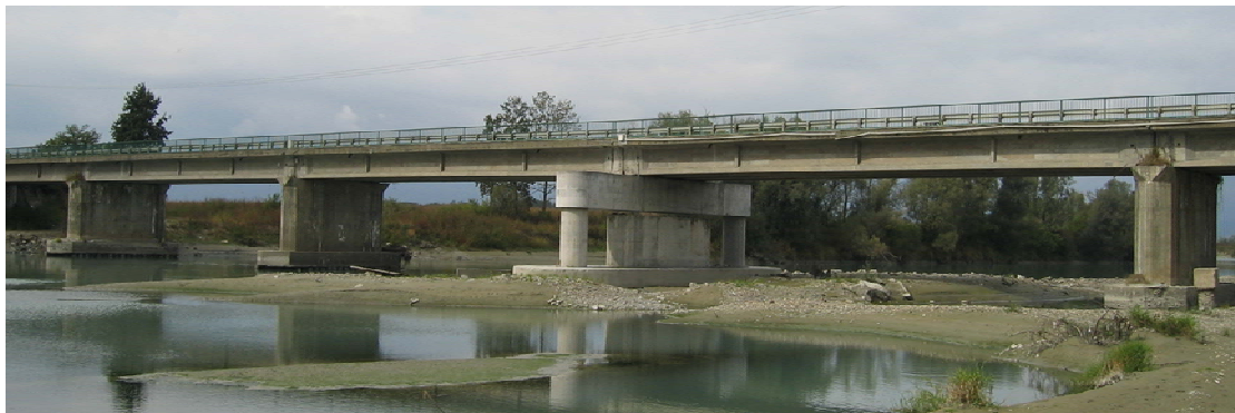
Figure 3 The bridge after retrofitting of pier P2 (Downstream view from North)
