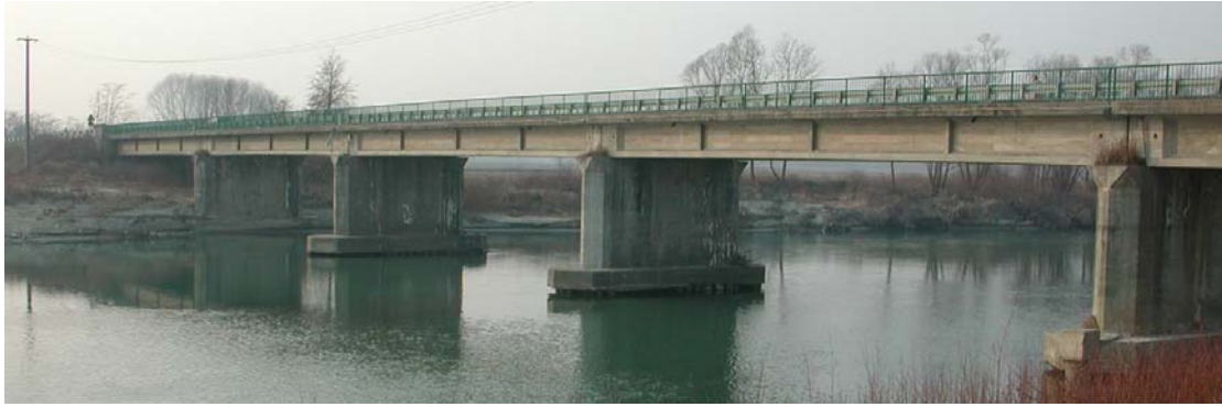
Figure 2 The bridge before retrofitting of pier P2 (Downstream view from North)
