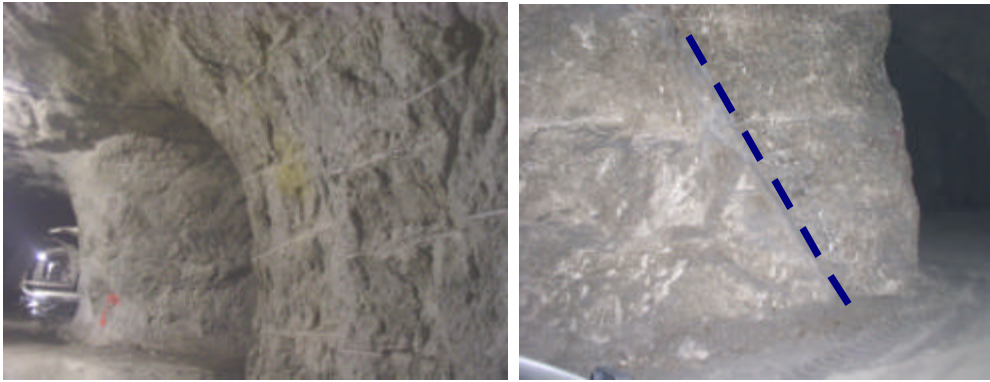
Figure 4. On the left, a room and pillar mine, excavated by blasting. On the right, a main transversal joint in a pillar.
