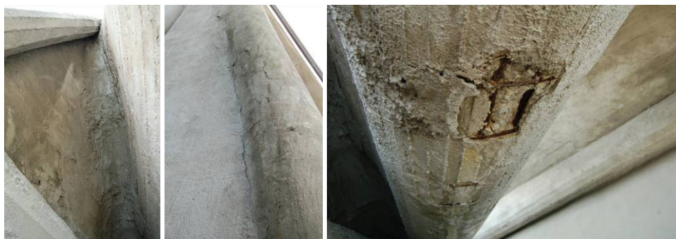
Fig. 15: present status of the building: a) internal point of extreme curvature of a vault, b, c) bar cover degradation.
