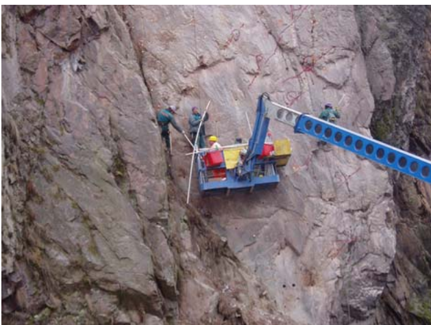
Fig. 11. Charging phase using a mobile platform. The charges were pre-prepared inside a PVC pipe to facilitate ease of placement into the drill holes.
