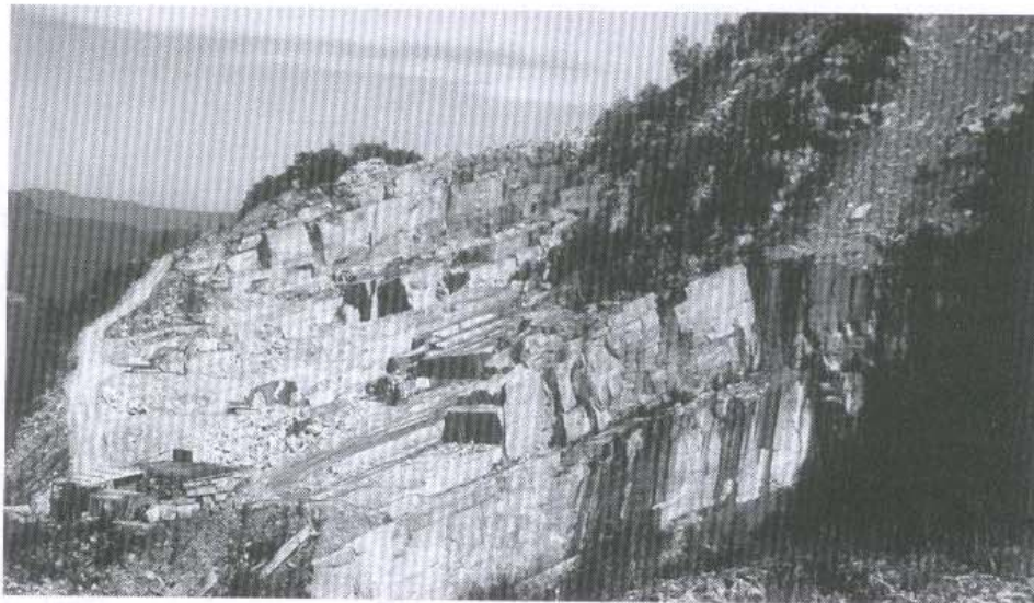
Fig. 2. Ornamental stone quarry with detritic and colluvial overburden.
