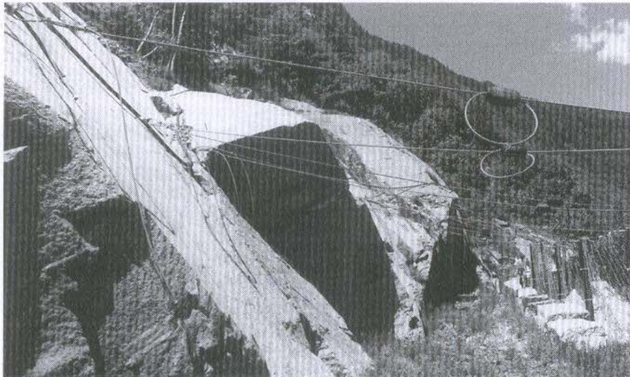
Fig. 4. Protection at the top of a geiss quarry with fences.
