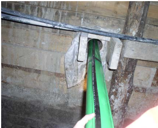
Figure 12. Detail of the installation of the asymmetric casing along a transversal drift in the Rodoretto mine for a length of 26m
