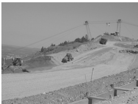
Figure 4. The earth-moving organization in the upper floor of the dump. On the right, a particular of the loading operation of one bucket of the ropeway.
