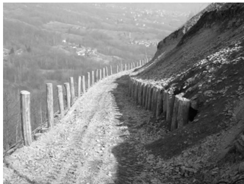
Figure 3. On the left, The reshaping of the upper part of the dump: the benches and the draining works are well visible. On the right, the berms created in the central part of the slope, to stabilize the dump body and intercept the run-off.
