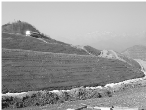
Figure 3. On the left, The reshaping of the upper part of the dump: the benches and the draining works are well visible. On the right, the berms created in the central part of the slope, to stabilize the dump body and intercept the run-off.
