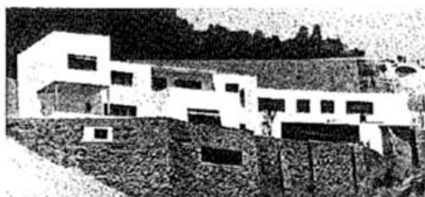
Bernard Rudofsky (?). Complete view of Oro house (designed by Rudofsky and Cosenza), 1937.
