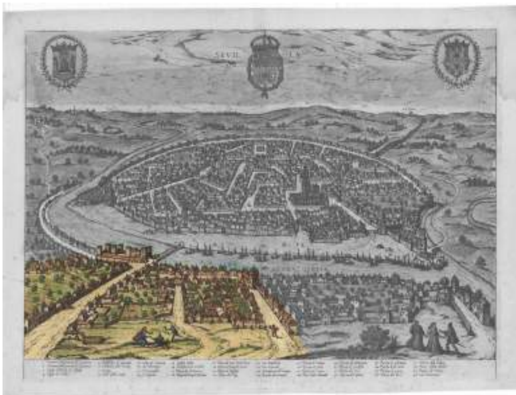
Figure 65: 1588, view of Seville by George Braun, included in the Atlas Civitates Orbis Terrarum . The area of Triana has been highlighted, including the Castle of San José and the bridge. © Instituto Geográfico Nacional, item number: 31-C-16. 267
