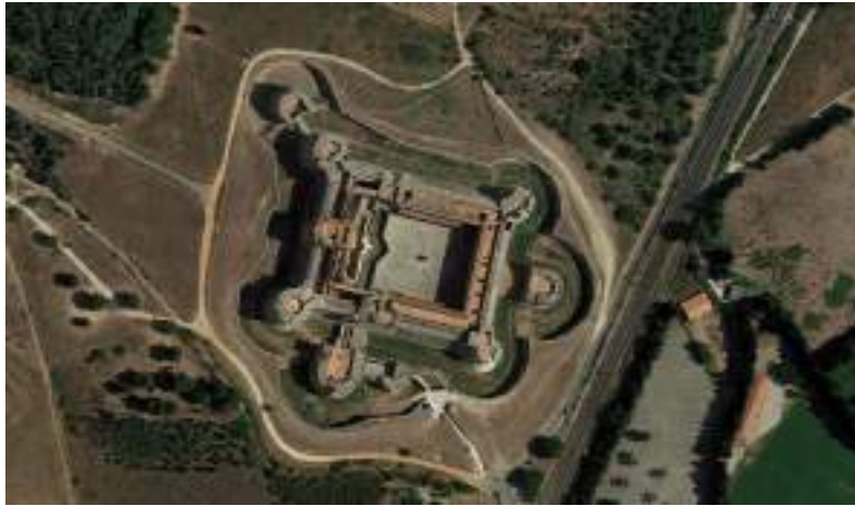
Figure 100: Satellite view of Salses Fortress, Roussillon, France. Its layout was modified by Ramiro López in 1496 by order of king Ferdinand II of Aragon. The east and south bastions were added at that point to the pre-existent fortress. © Google Earth
