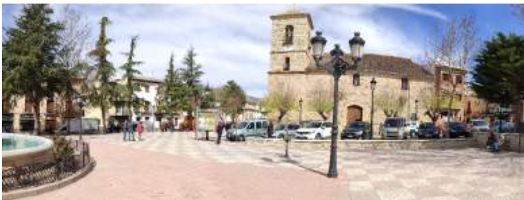
Figure 184: The main square of Campillo de Arenas, named Plaza de Andalucía. The church of Nuestra Señora de la Encarnación faces the square with its long side, in a similar fashion to Valdepeñas. The city hall is located in a white building, visible on this picture on the left of the church. In this way, the church and the council house face each other, forming a secondary public space annex to the main square. © Manuel Sánchez García, 2020.
