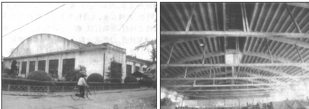
Fig. 3-16 Exterior and interior of the hangar in the Xigong (Source: Luoyang Jianzhuzhi )
