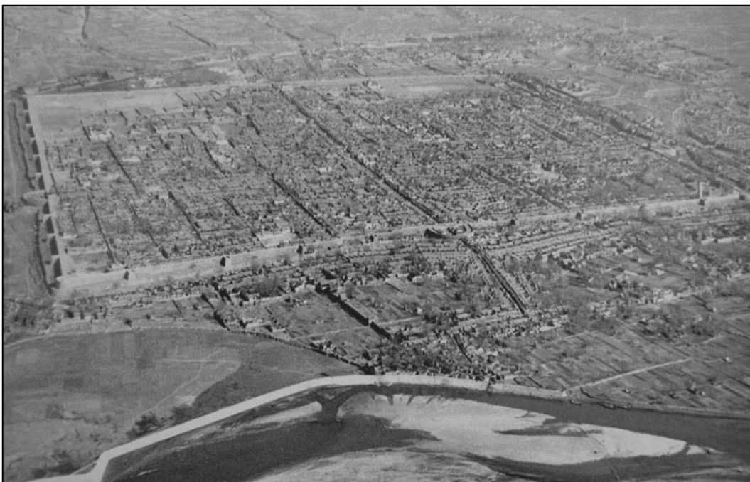
Fig. 2-8 The aerial photography of Luoyang in 1930s (Source: https://m.thepaper.cn/newsDetail_forward_1528201?bdchannel= )
