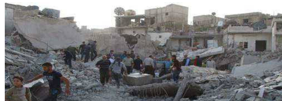
Fig.8. Destroyed concrete buildings in Aleppo, Syria (Aljazeera, 2016).
