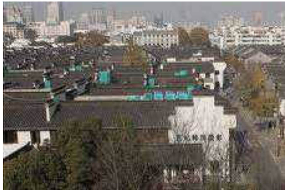
Fig.5. Identification of roof air conditioning.
