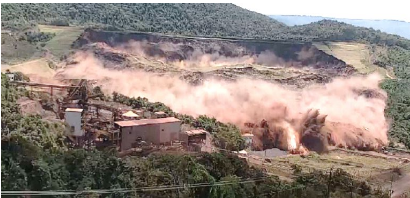
Fig. 1: The collapse of Feijão tailing dam - Brazil – 2019 ([8]).
