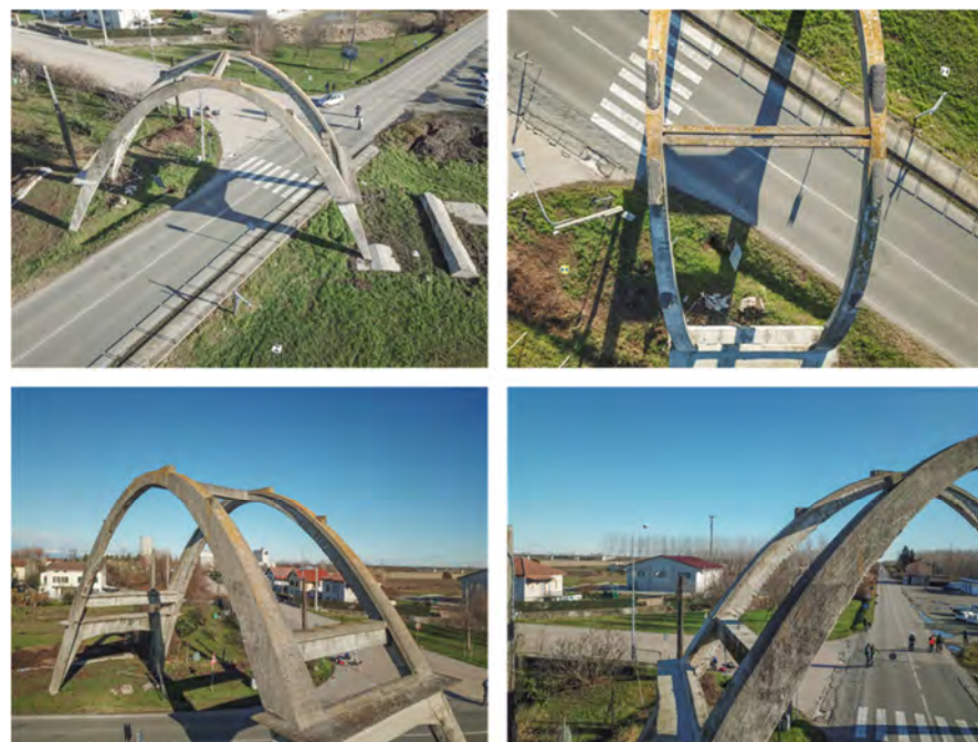
Figure 4. Digital images acquired from an aerial perspective using the micro UAV system, which enabled the acquisition of the extrados and the higher surfaces of the concrete arch.
